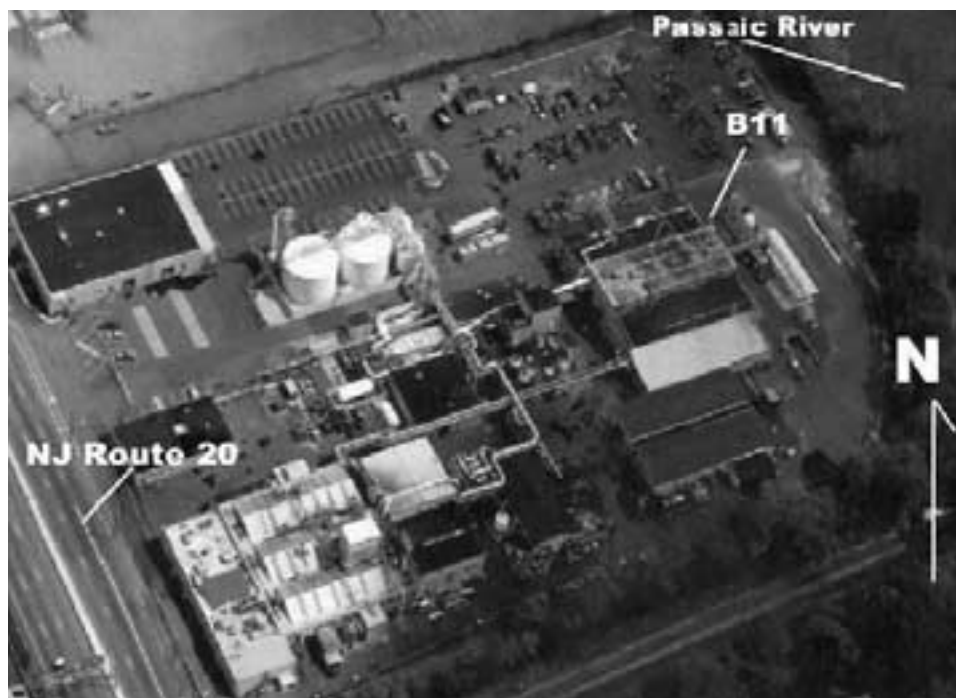
Figure 1: Aerial View of the Paterson Plant
