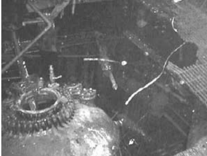
Figure 12: Post-accident Photo of the Kettle
