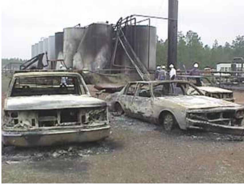
Figure 7. Damaged Vehicles and Storage Tanks
